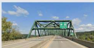
WV527 over Ohio River (Truss)
