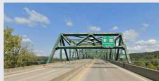
WV527 over Ohio River (Truss)
