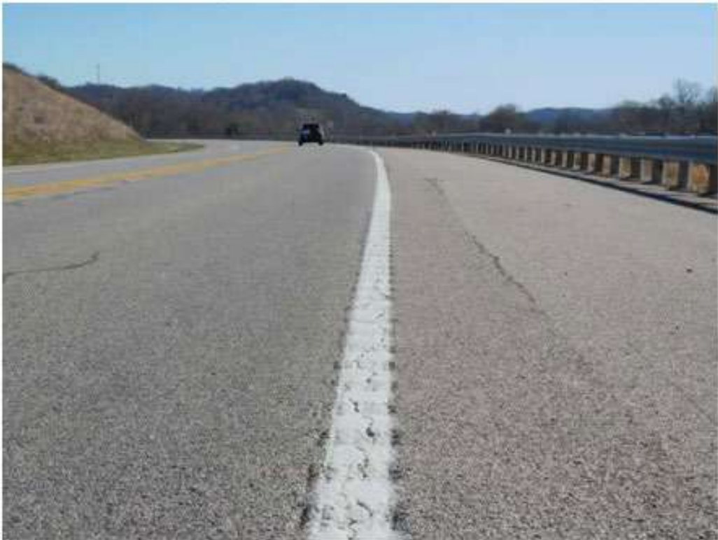
Figure 13 OH SR 7 Between OH SR-775 and Athalia (North and East of Proctorville)
