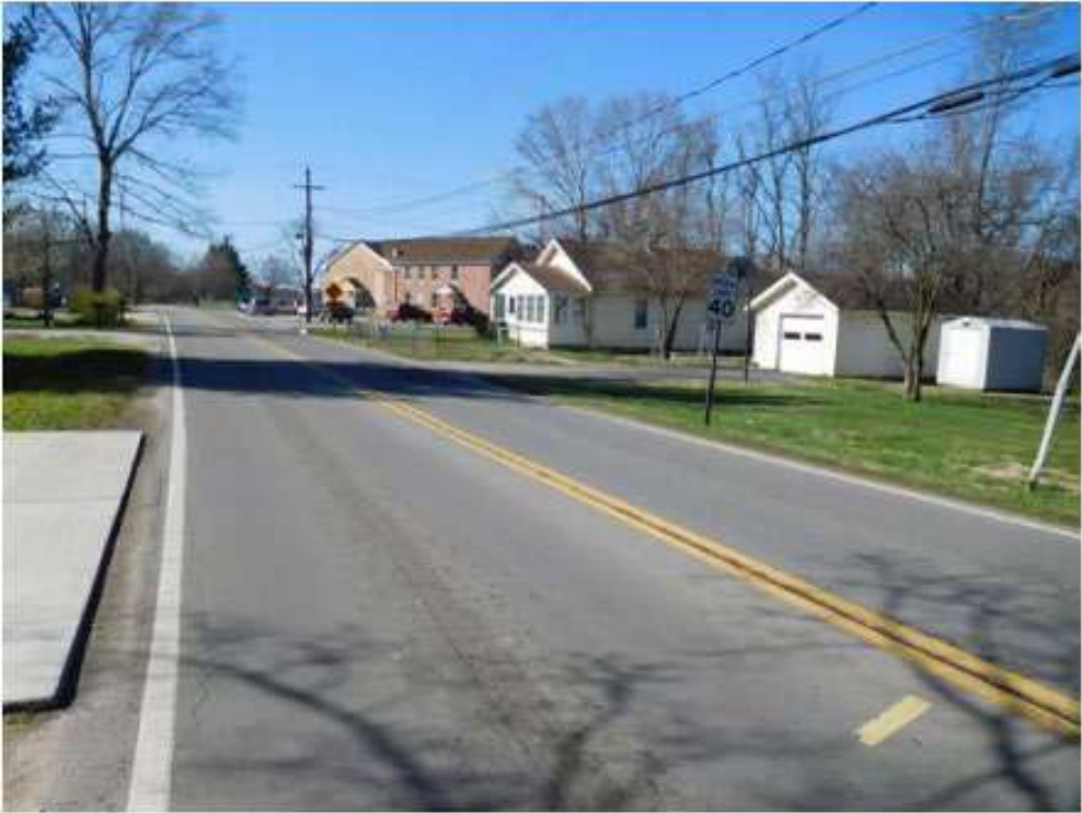
Figure 15 SR-411 between Cedar Street and Beulah Lane (Proctorville)
