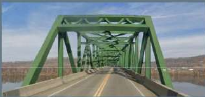
US 52 over Ohio River (Truss)
