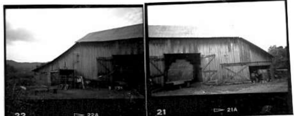
BARN: NORTH ELEVATION
