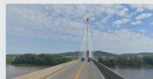
WV106 over Ohio River (Cable-Stayed)
