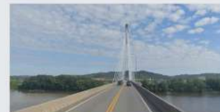
WV106 over Ohio River (Cable-Stayed)
