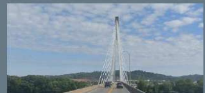
WV106 over Ohio River (Cable-Stayed)
