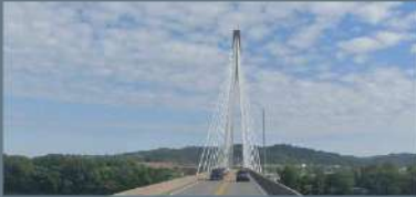
WV106 over Ohio River (Cable-Stayed)
