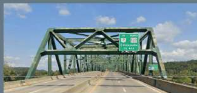
WV527 over Ohio River (Truss)
