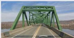
US 52 over Ohio River (Truss)
