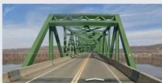
US 52 over Ohio River (Truss)
