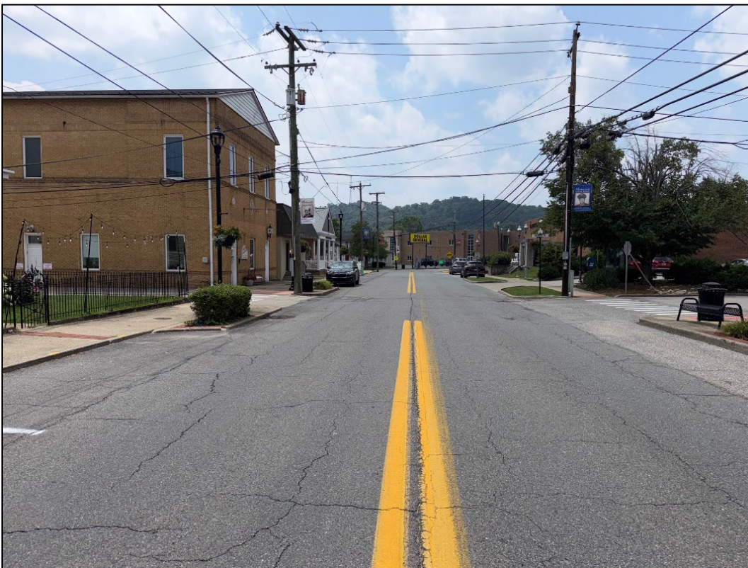
Figure 4: Central Avenue – Looking South
