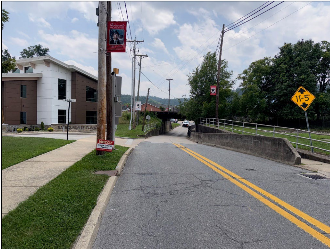
Figure 2: Looking South at CSX Underpass
